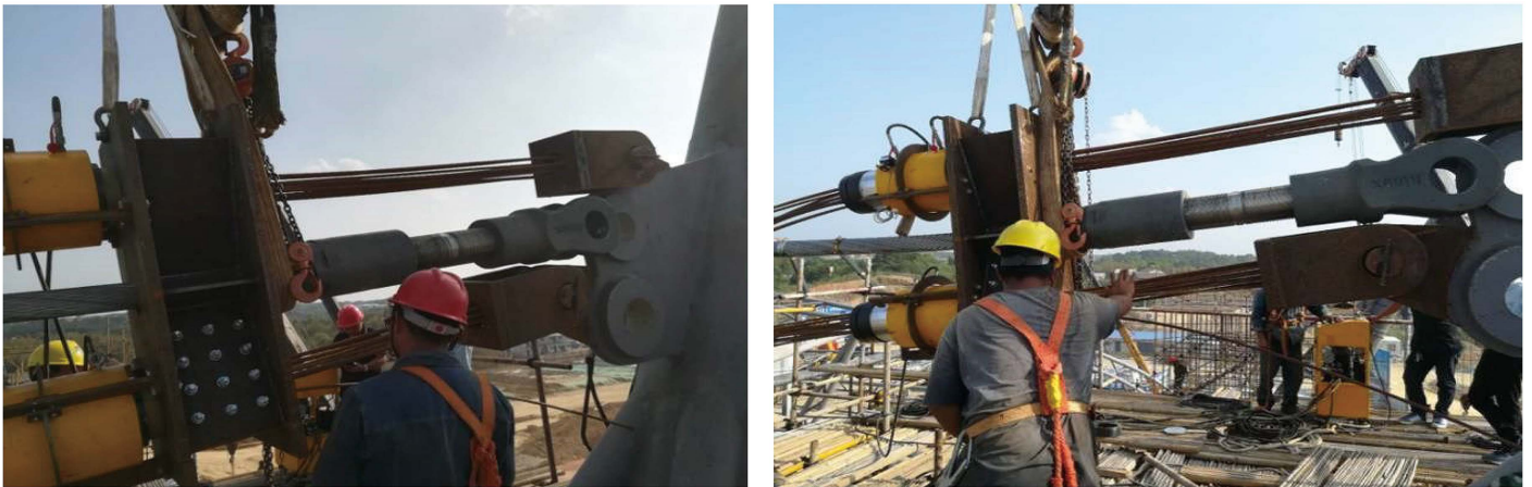
Fig. 6. Tensioning the suspension cables.
