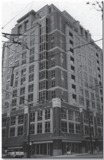
Fig. 12 Picture of the investigated building.
