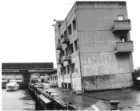
(a) Failure pattern of a pile-supported building, photo courtesy K. Tokimatsu
